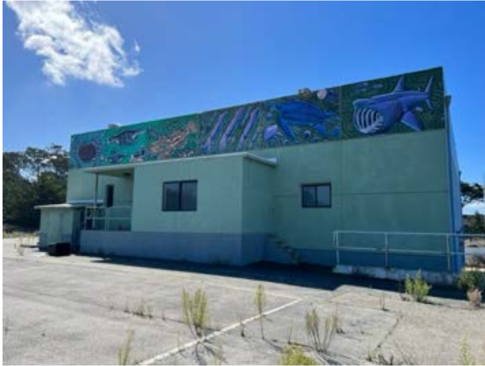
Photograph 3: View looking south at the rear of the building.
