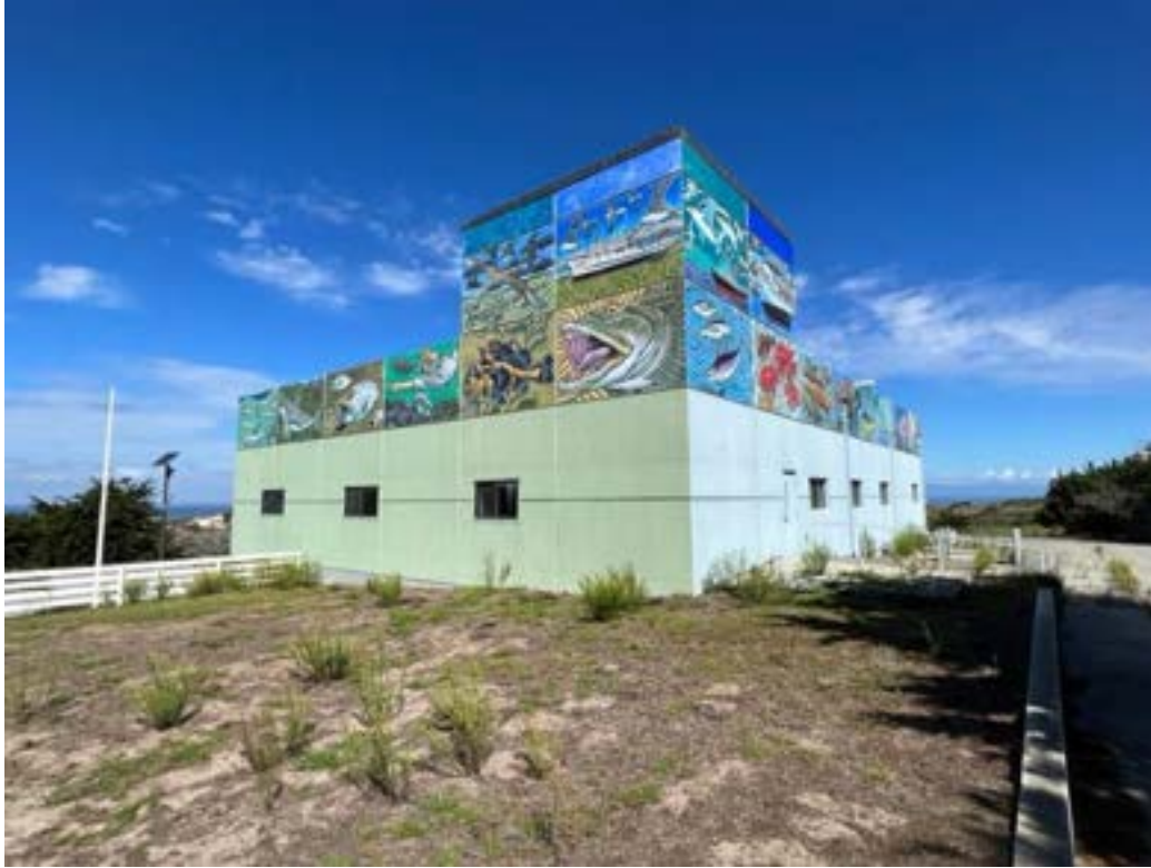
Figure 2: View looking northwest at the southeast elevation of the building.
