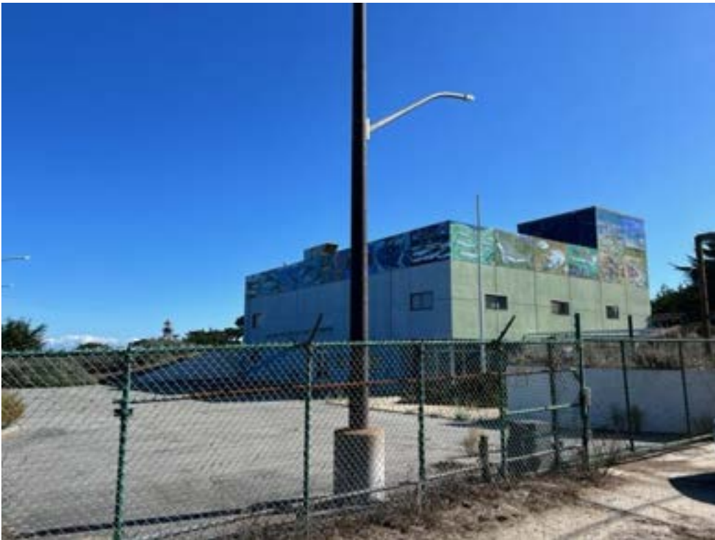
Figure 3: View looking northeast at the southwest elevation of the building.
