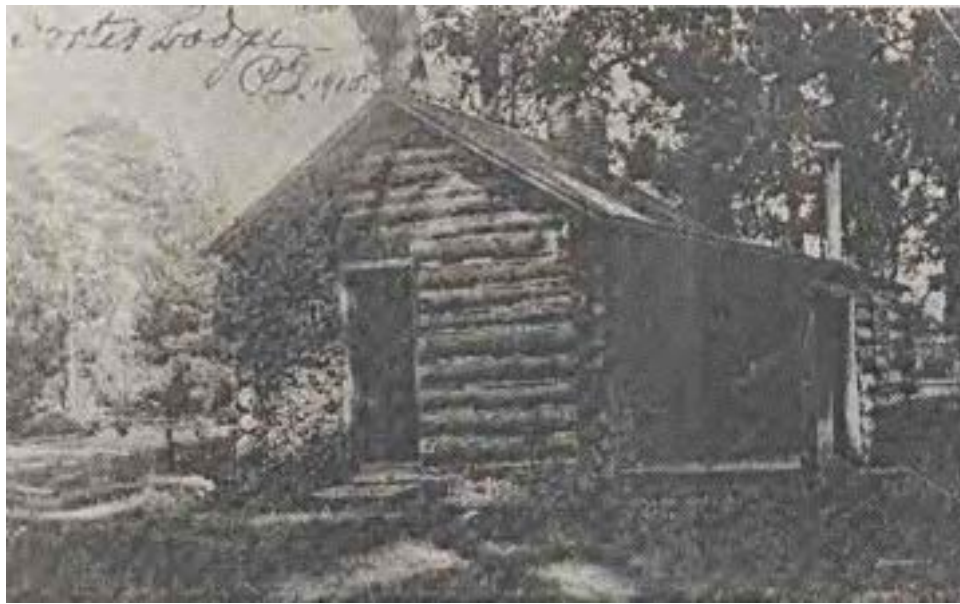
Porter Lodge at 301 Alder, originally constructed for Mrs. Clara E. Curtis. Photo 1910. (Heritage Society of Pacific Grove, Board & Batten , February/March 2000)
