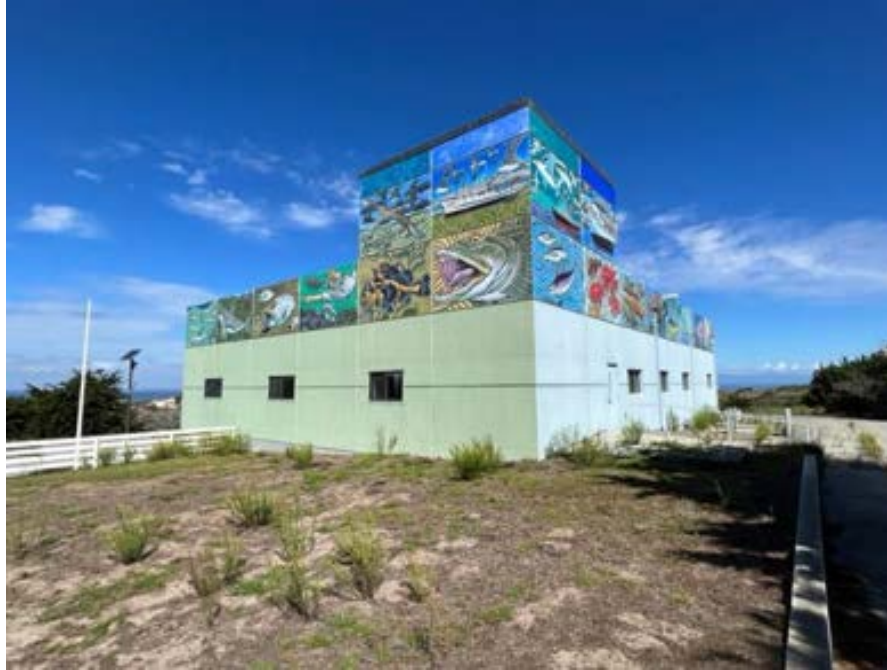
Photograph 1: View looking northwest at the building from Lighthouse Avenue.
