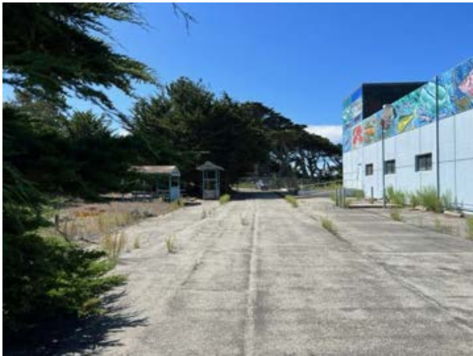
Photograph 4: View looking south at the east elevation of the building.
