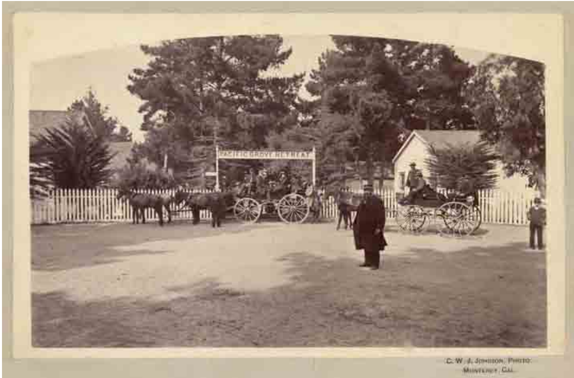
Retreat office and stile gate entrance at Lighthouse and Grand avenues, 1885. Joseph Oscar Johnson (lower right) was hired by Jacks as Superintendent of the Retreat, and was responsible for greeting visitors at the gate. (Photo by C.W.J. Johnson. California State Library)
