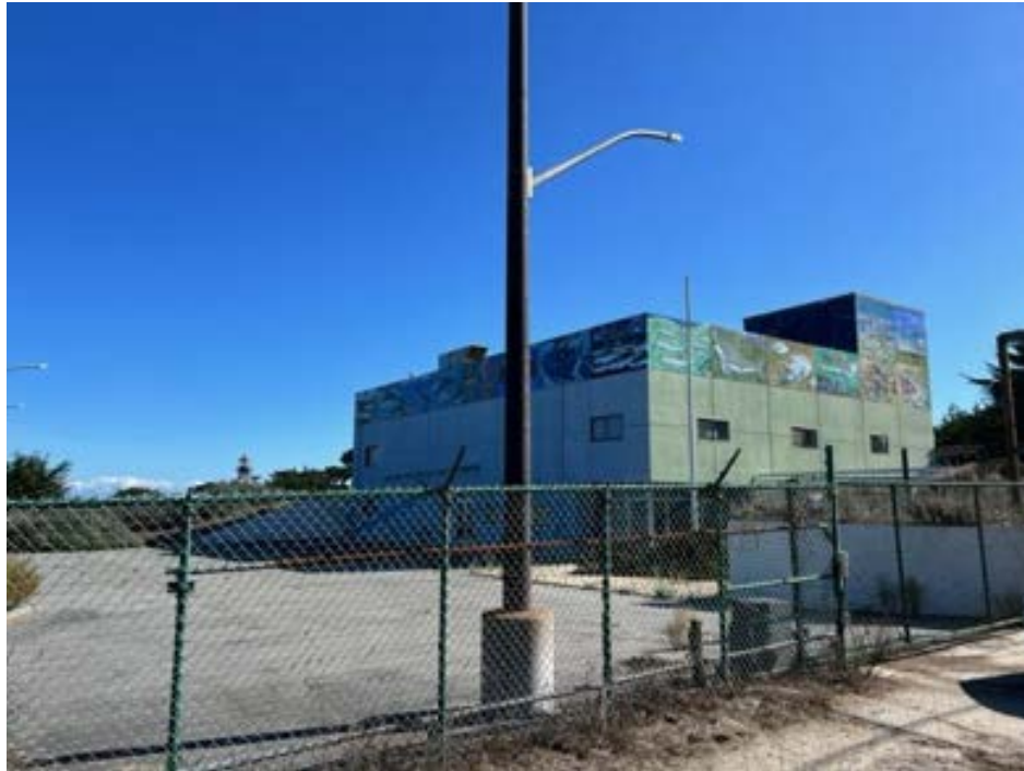
Photograph 5: View looking northeast at the southwest elevation of the building from Lighthouse Avenue.
