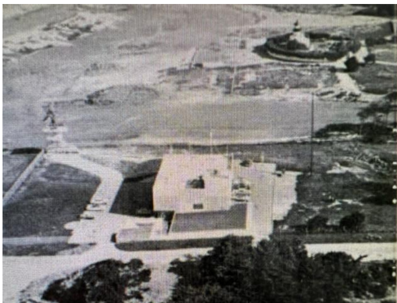
Figure 1: 1961 photograph of the Point Pinos Naval Air Intercept Training Facility looking north. The radar installation can be seen on the top left corner of the photograph. Note the single window on the south facing wall of the building (All Hands Naval Bulletin 1961).
