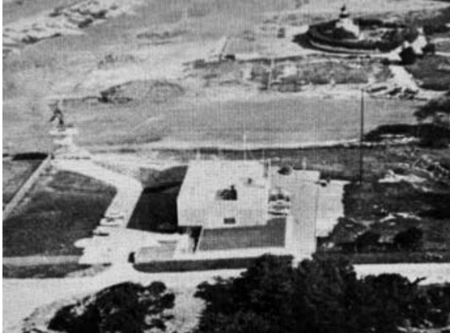
The Point Pinos Naval Air Intercept Training Facility. Source: All Hands Naval Bulletin, March 1961
