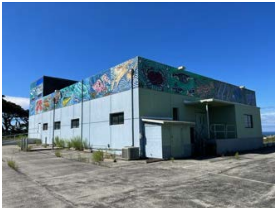
Photograph 2: View looking southwest at the building. The bump-outs in the rear are built of concrete block and are later additions.
